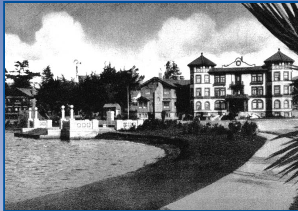
Historic Postcard showing stairs and lights to be replaced
