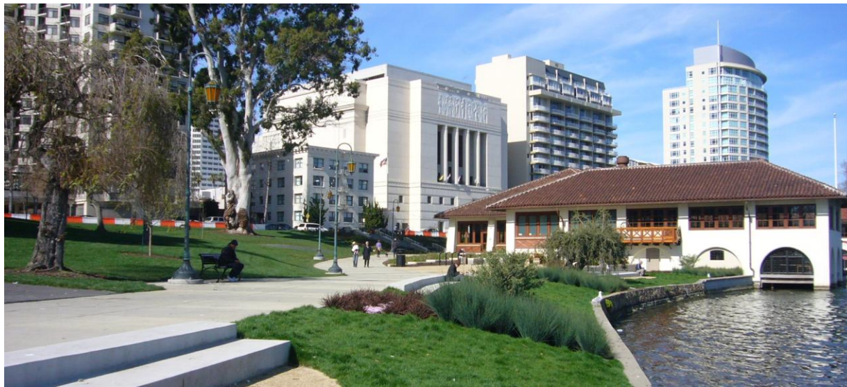
After project improvements, with multi-use path
