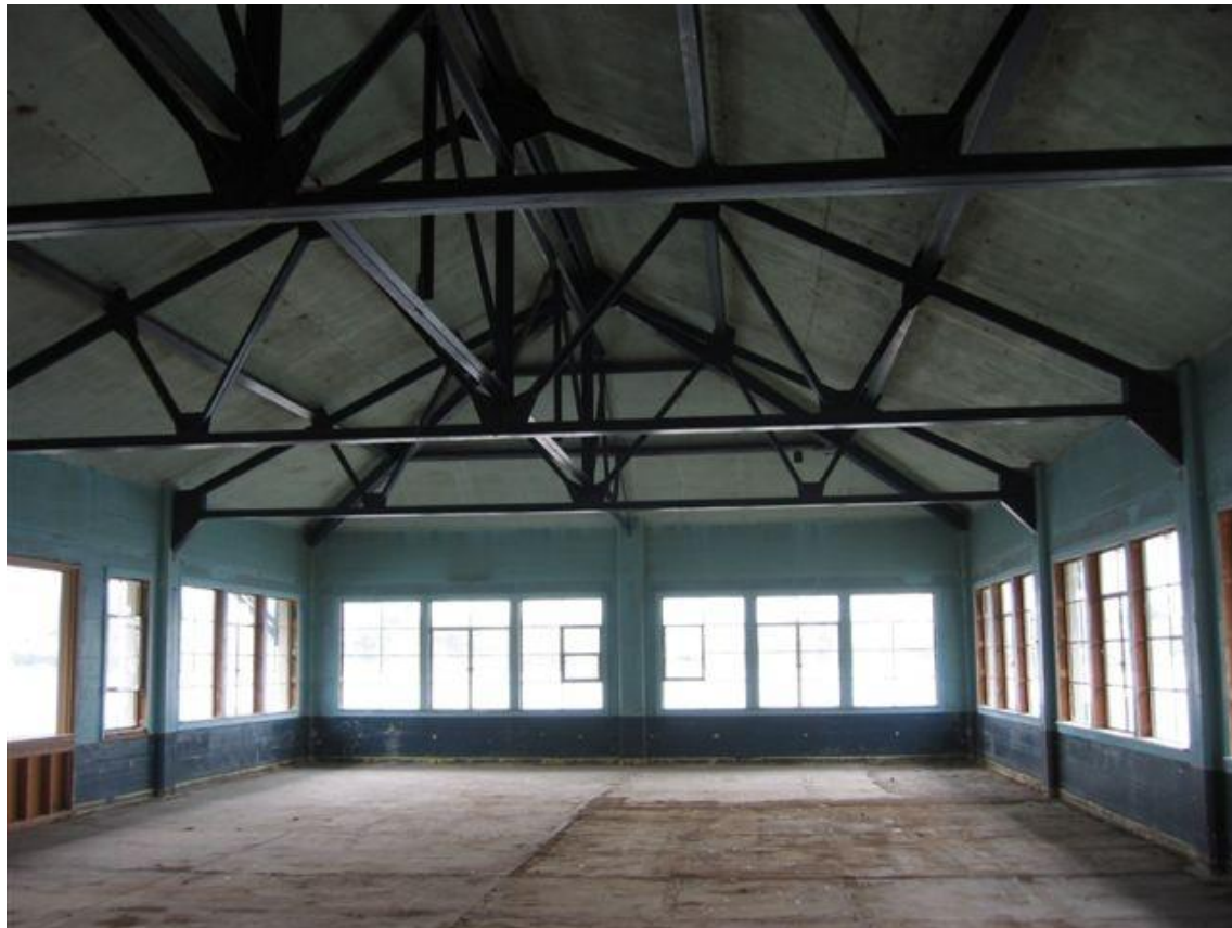
South wing after demolition of ceiling and interior walls
