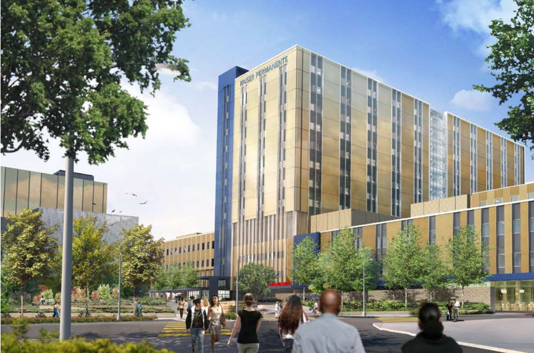
View from Piedmont Avenue looking west
