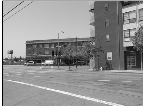
Photo V.A-2: View southwest from the project site, across Adeline Street and San Pablo Avenue.
