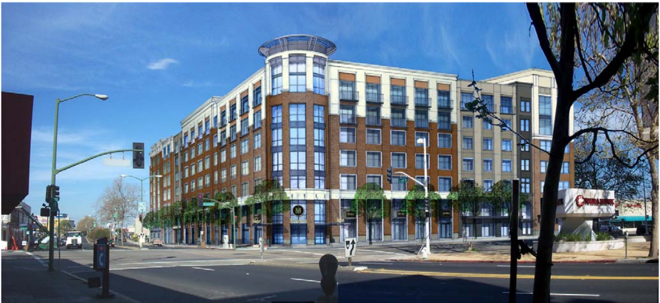
A. Proposed view of the site from the intersection of Broadway and West Grand Avenue looking northwest.
