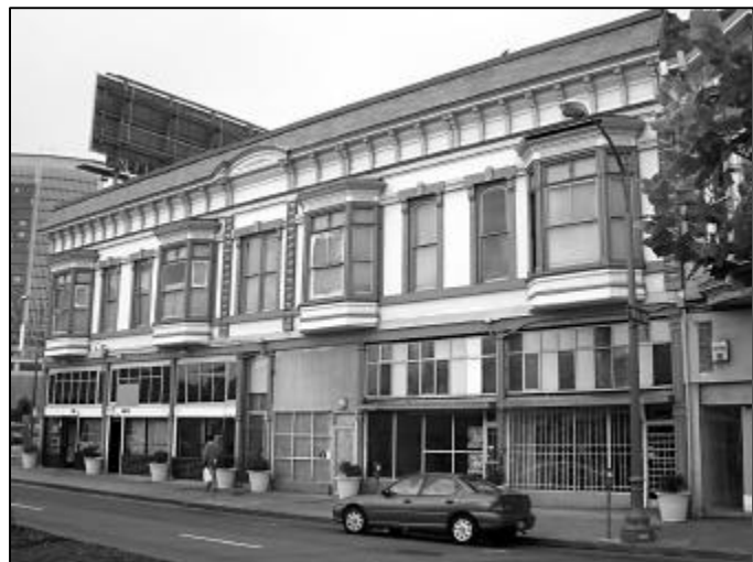
A portion of the 19 th and San Pablo Commercial District
