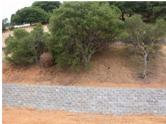
Photo 2. Photo shows the cut slope below the oak trees where mulch and water are still required.
